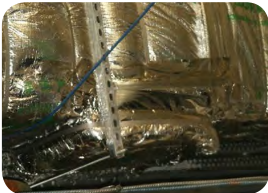
Insulation cover must be easily removable Banding over doors should be avoided
